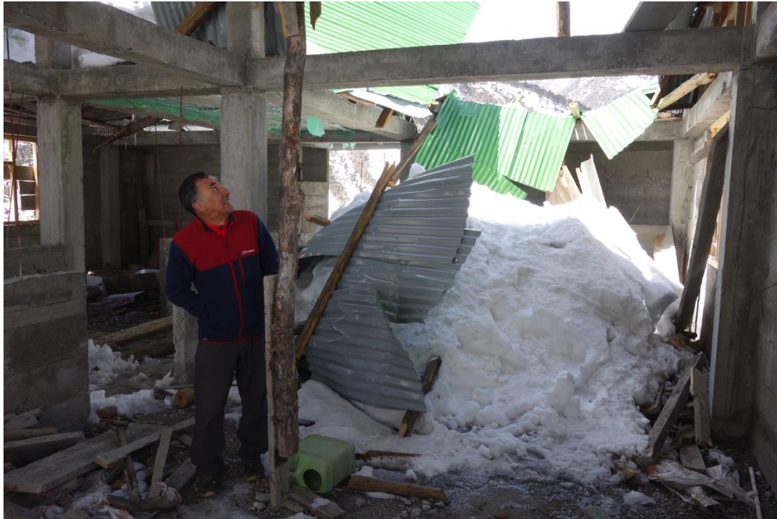
Winter snow damage at our hotel in Tangu
