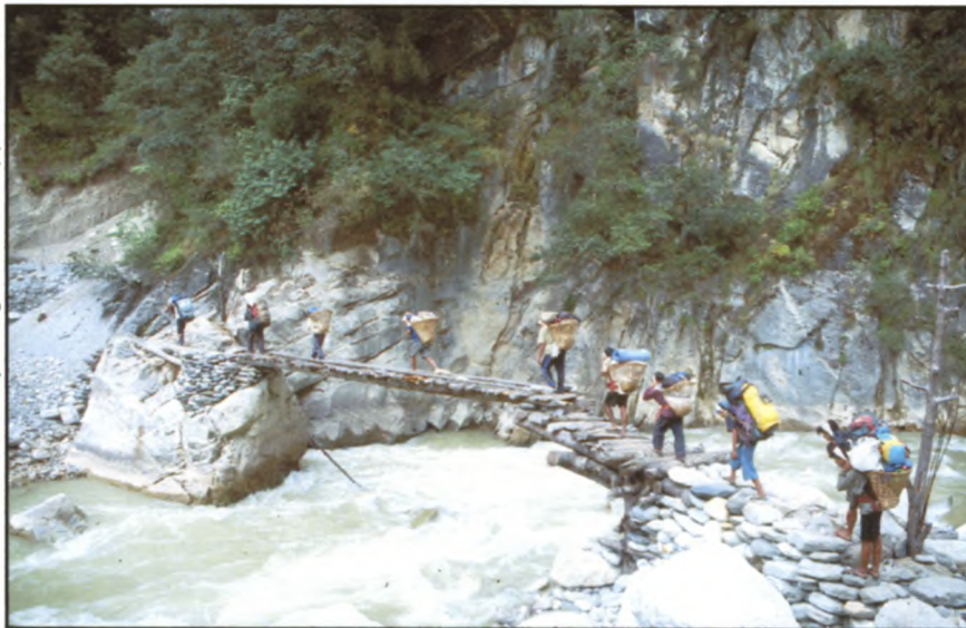
One of the many bridges on the approach
