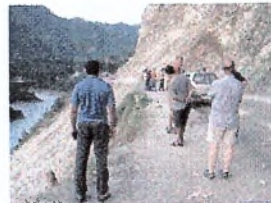
One of many landslides
