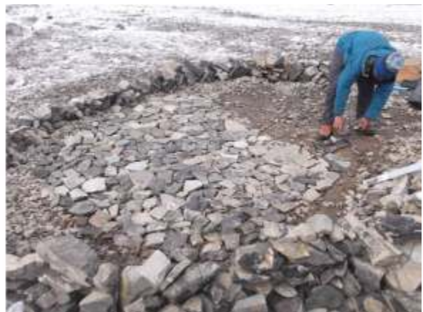
Alek building a level platform (R. Kernan)
