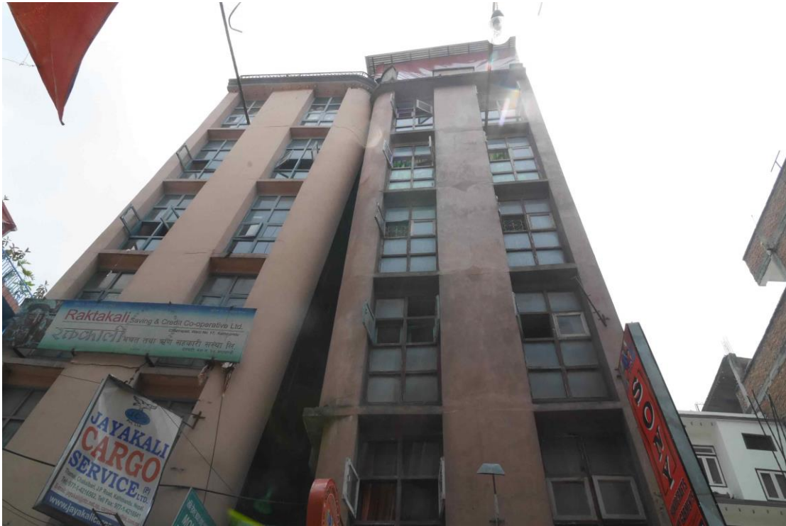
Building toppled into each other in Kathmandu
