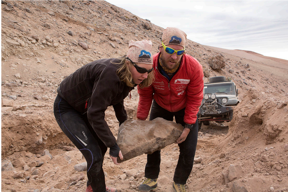
Figure 21. Suzie and Max (and Pedro!) rebuild the road up to Mt Copiapo.
