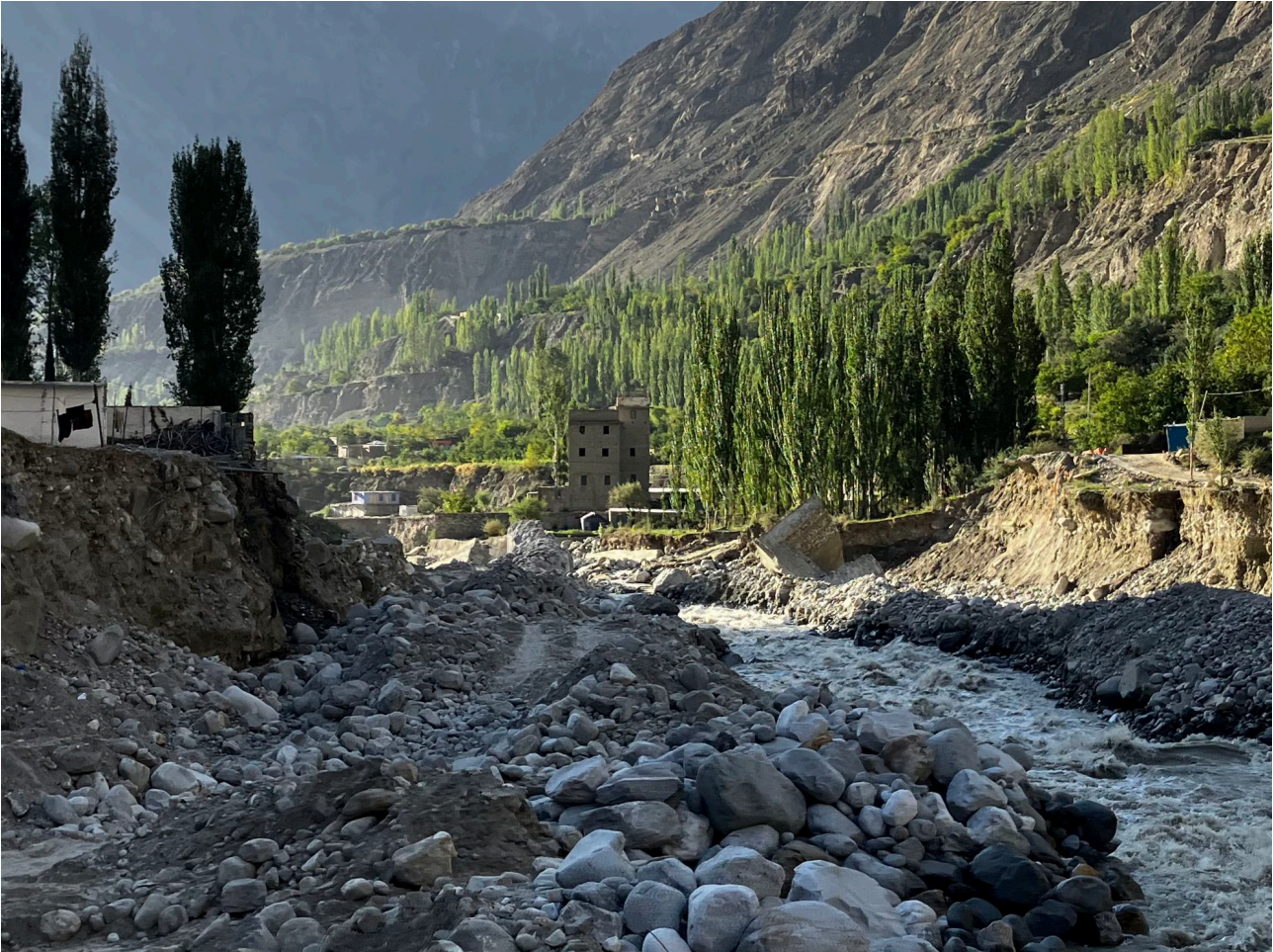
What's left of the Hassanabad Bridge and the Karakoram Highway, Hunza
